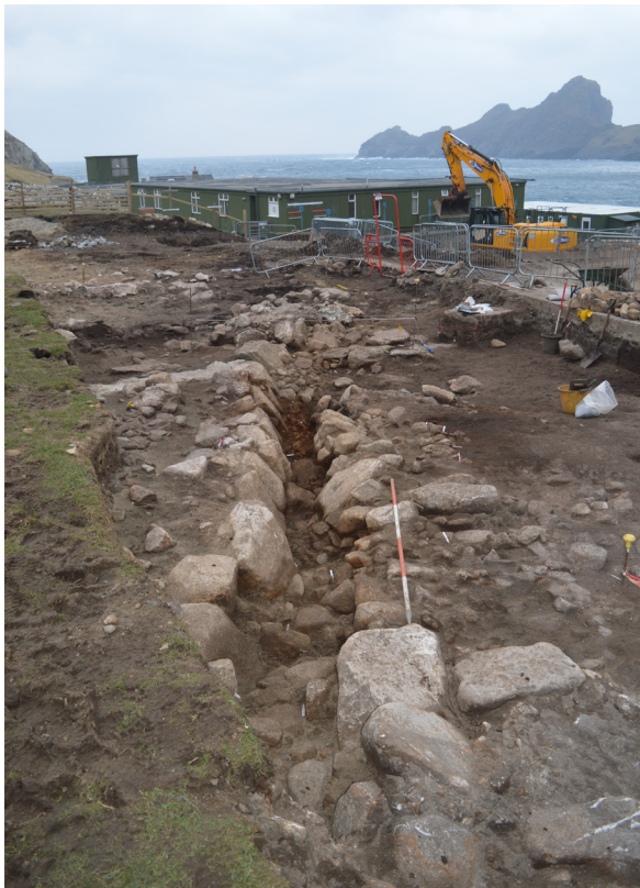
Plate 5: General view of the channel. Taken from the north-west.
