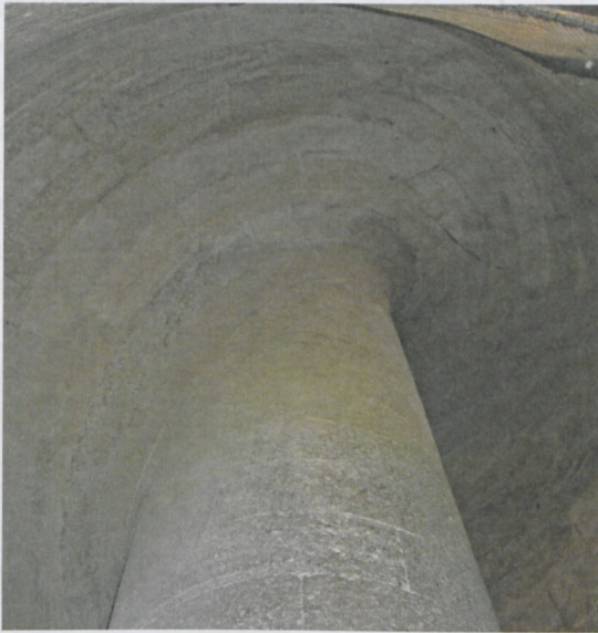
FIG. 8 – Spiral stair of the abbey church of St. Gilles, vault.
