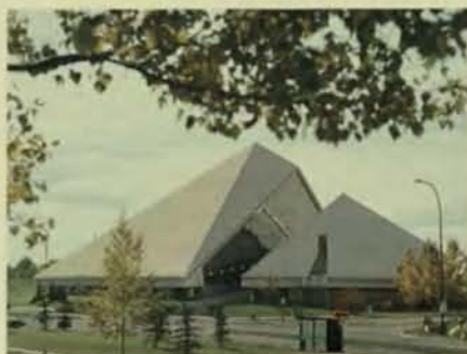
The Calgary Public Library in Calgary, Alberta is one of AWI's fabricated steel buildings.
