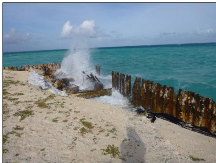
Figure 3-9 Seawall in 2013 in Calm Seas (FWS photo credit)
