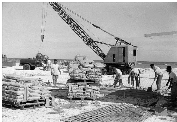
Figure 3-8 Constructing Tern 1942 (National Archives)
