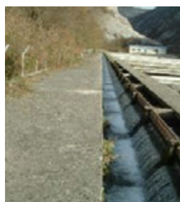
Outlet channel of tanks
