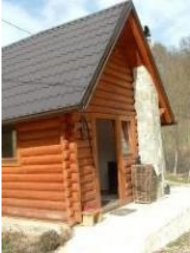
Office and guard house
