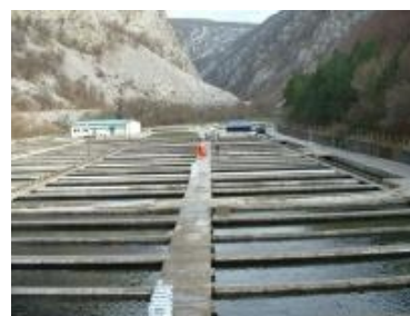
Tanks with total volume of 10 000 m 3
