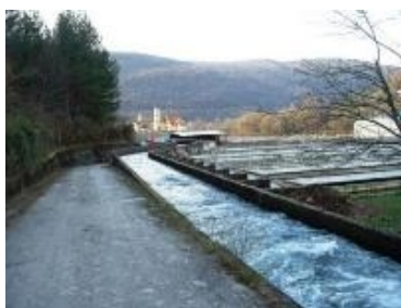
Inlet canal with 4 m 3 /sec water transferring capacity
