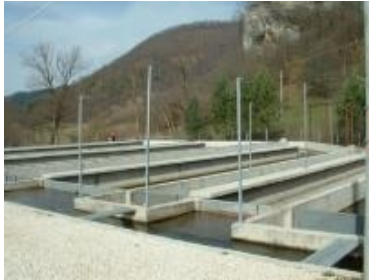
Inlet screens of fish tank
