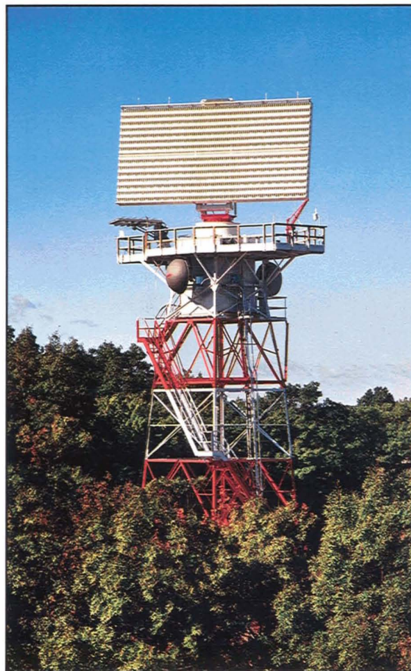
Fig. 1—UHF ultralow-sidelobe array antenna installed at Lincoln Laboratory.
