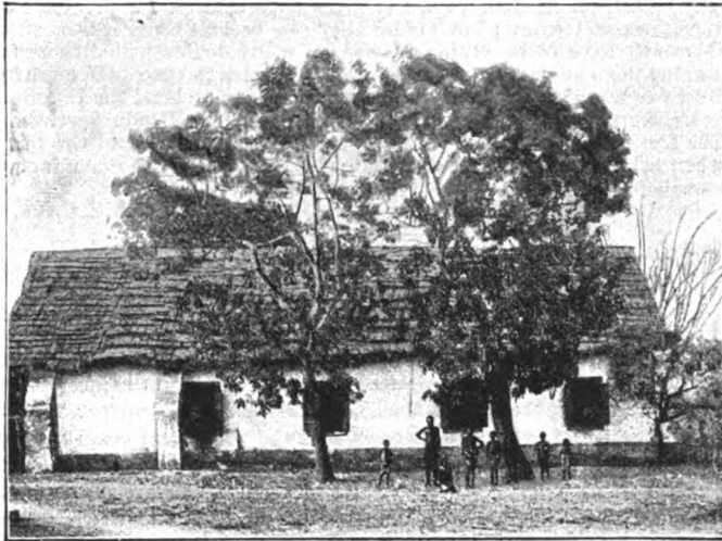
MR. REBMANN'S OLD HOUSE AT KISULUTINI, USED FOR A TIME AS A CHURCH.
