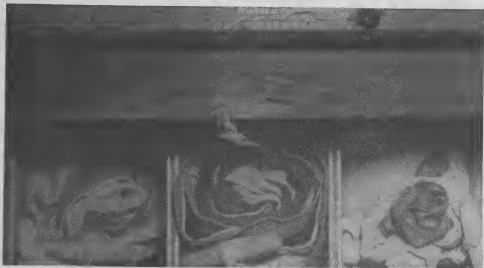
Shown above is the flag locker on the bridge of the lake tanker Boscan, illustrating ravages of termites.
