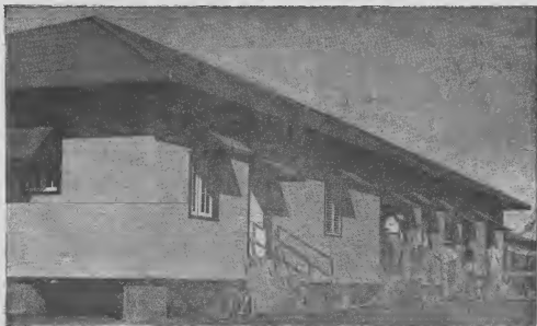
Shown above is the training building located at the old Garage site. The men seen leaving the building are members of a class in refining fundamentals, taught by John Preston.
