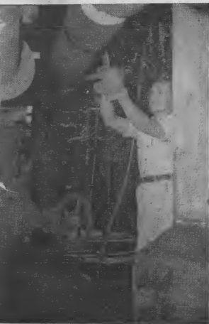
Mathias Camacho, Levelman, adjusts backtrap on No. 6 Combination Unit (in other words makes an adjustment to control the liquid level in the bubble tower). For pictures of other levelmen and the work they do, see page 9.
