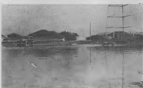
Shown above is a view of the lake that washed motorists' wheels and provided sport for children in front of the Colony Commissary after the recent heavy rain. The depth of the water can be seen at right, where one of the boys is sitting on a wagon that is completely covered.
