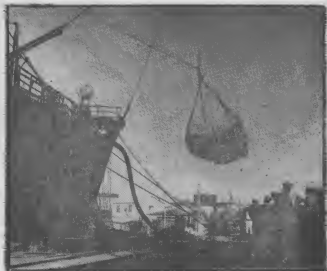
Conventional sling unloading is shown at right. Most cargo is unloaded by this method.
