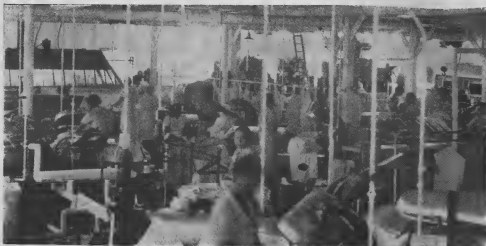
Shown above is a view of the pressing department of the Laundry. The numerous pipes visible carry compressed air and steam. In the left background is a new canopy that takes heat from the flatwork ironers
