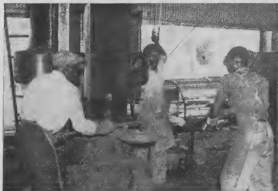
At left, blacksmiths Charles Newton and George Hemstrack swing sledges on a red-hot turnbuckle for the drydock, while Simon Richardson manages the controls of the machine that holds it firm.
