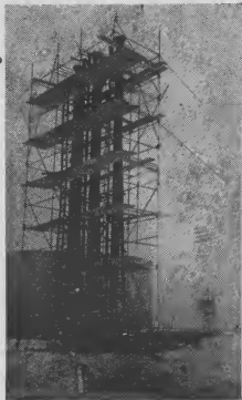
Above, left, is shown the submarine pipe bank nearly completed for launching. The horizontal portion will be buried under the floor of the harbor in a trench dredged across the west entrance channel, and ships will pass through the 500-foot space between the "risers". Right, at top, hundreds of tons of material are being transported to the site on barges. Being swung aboard is a pile with "legs", or bolted-on cleats that increase the resistance of the pile. Below, the bucket dredge chews out a trench on the harbor floor for the pipelines.
