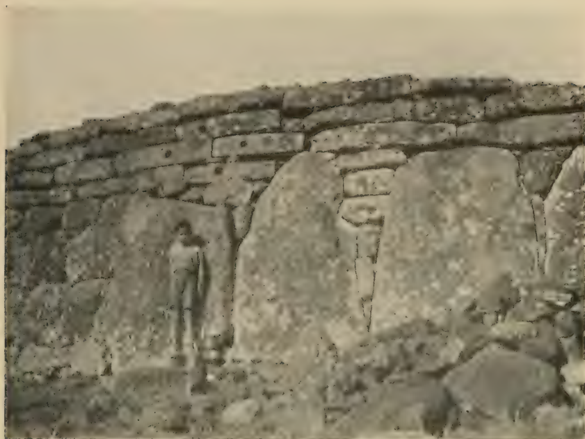
1. SEAWARD FACADE OF AHU (BURIAL PLATFORM) TE-PEU. Notice in the structure pitted slabs taken from house foundations.
