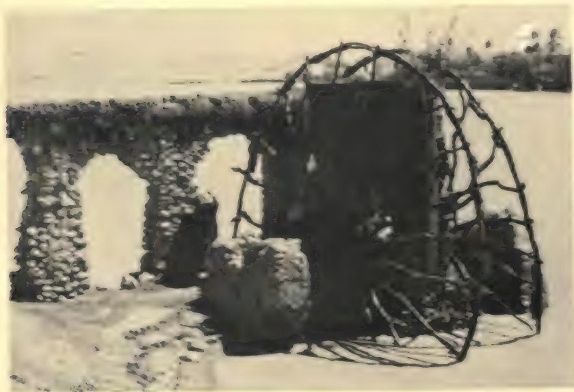
WATER-WHEEL AT HADITHA
