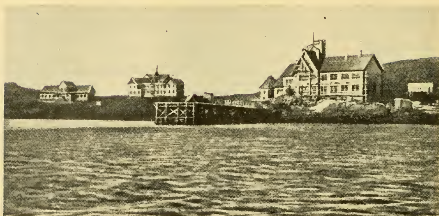
FIG. 50. Murman Biological Station of the Academy of Sciences of the U.S.S.R. in the Dal'naya Zelenetskaya Guba on the Murman Peninsula coast (1938).
