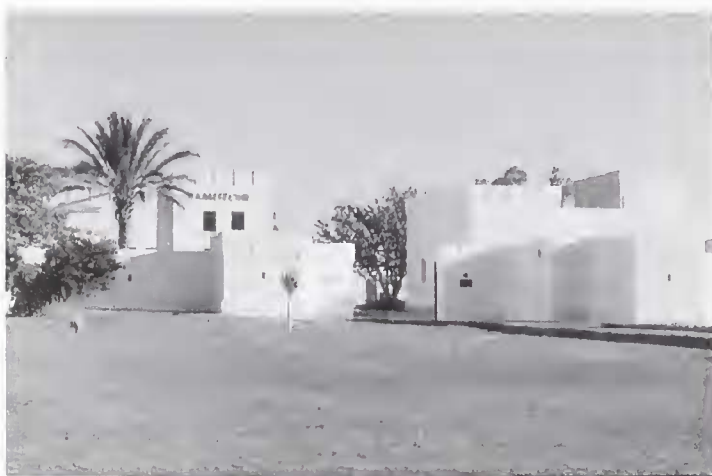
Fig. 27: Namutoni Fort, northern Namibia. This fort was erected in 1903, during the brief period of German colonial rule (1884–1915) and now serves as a tourist camp in Etosha National Park. Photo by the author.
