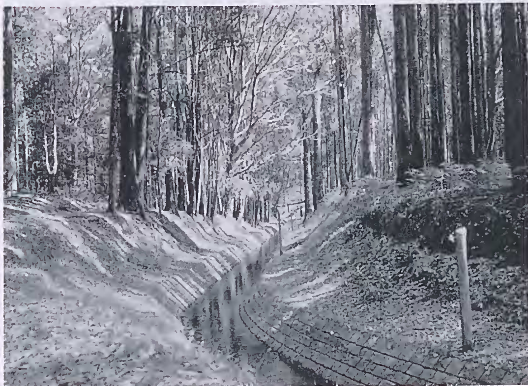
Fig. 9. Aqueduct from Wallaby Creek to the Great Divide at altitude of 510 m.
