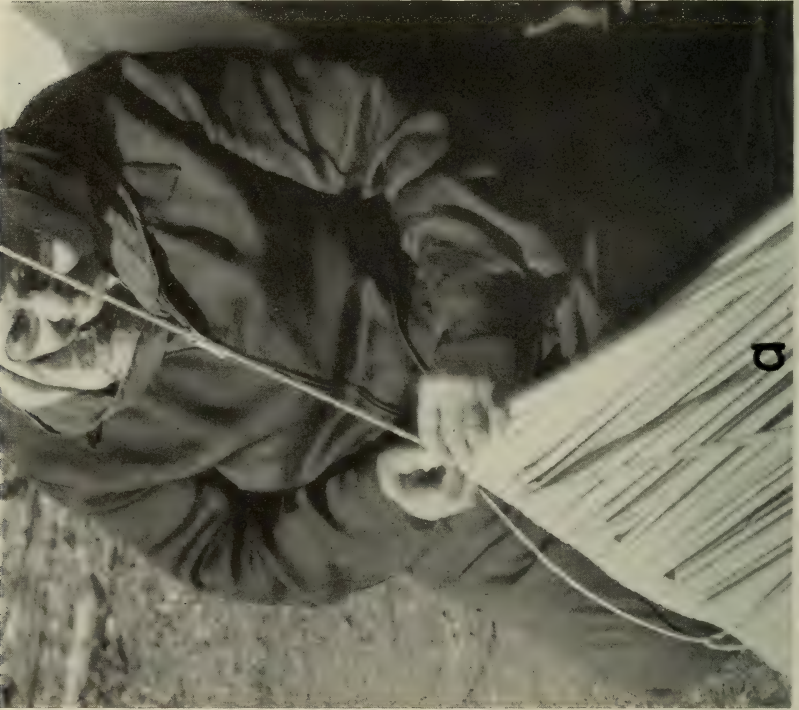
Making a cattail-mat wigwam cover. a , Mrs. Wadena tying a leaf into the selvage. b , Beginning the sewing of the mat.
