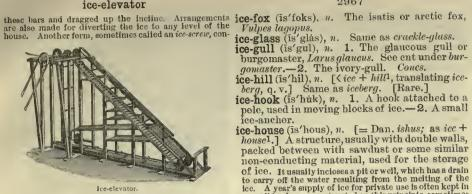
sists of an inclined plane in the ferm of a spiral. In the weil of the spiral is an upright shaft having radial arms; as the shaft revolves these engage the blocks of ice, and push them up the spiral incline to the ice-house.
