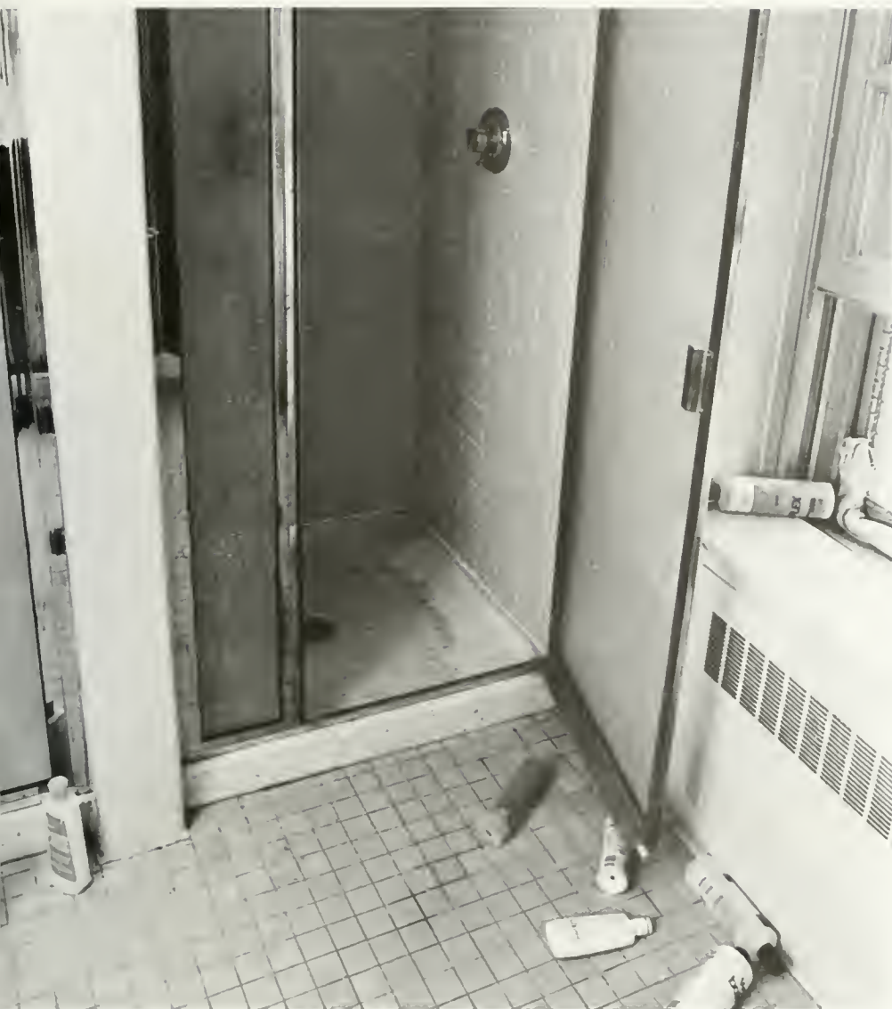
◀ Jefferson, under reconstruction since the fire in January 1983, opened for student occupation in January 1985. A passing scene shows the new hall showers which are, in many cases, nicer than the ones we have at home.
