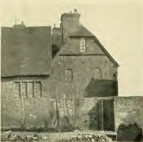
West side showing the blocked windows
