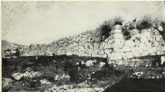
The old walls of an Italian town, made of large irregular blocks of stone such as Romulus might have used.
