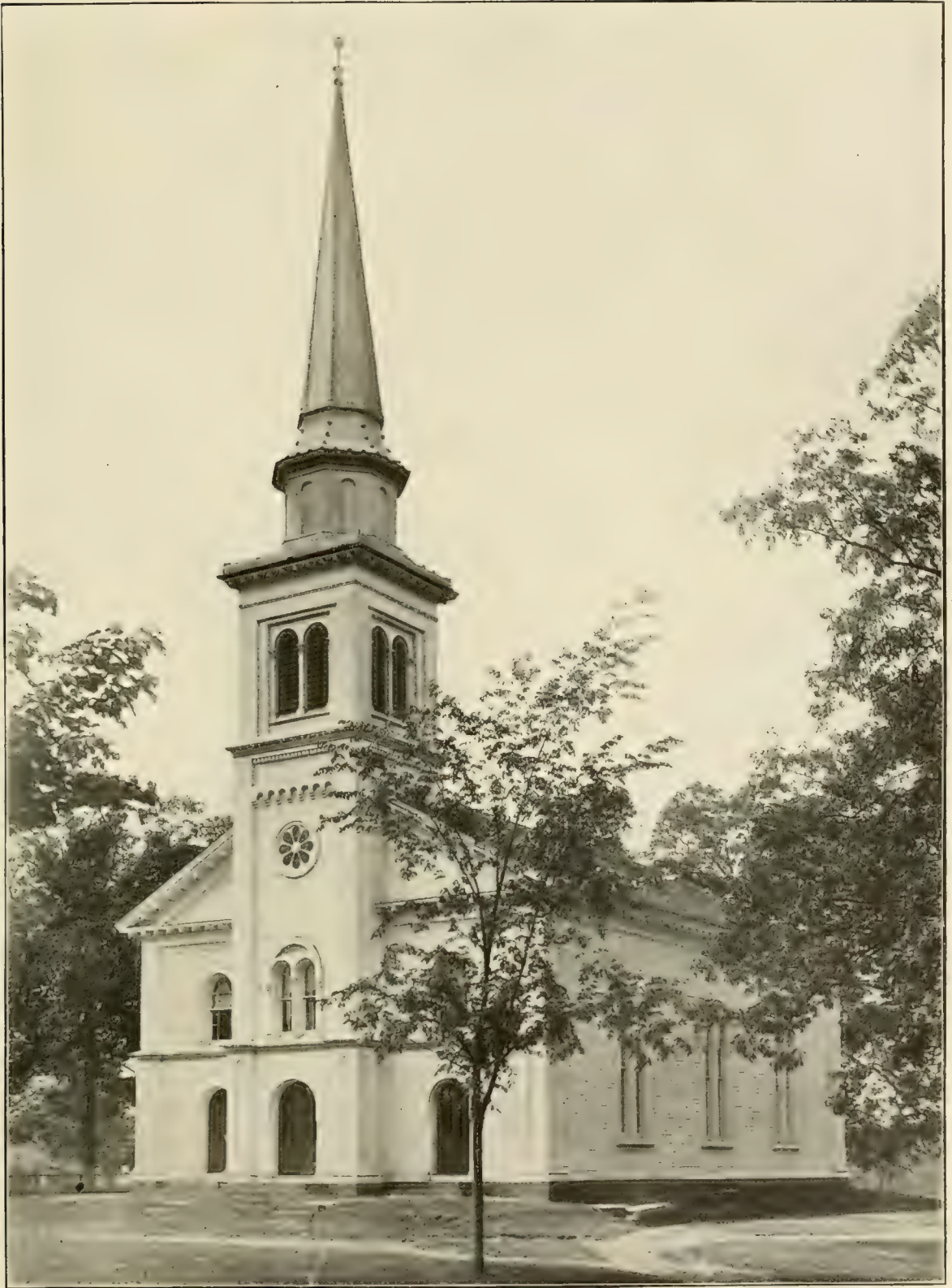
FIRST CONGREGATIONAL CHURCH, LUDLOW CENTER
