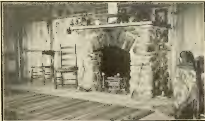
INTERIOR OF F. L. BURR'S BUNGALOW
