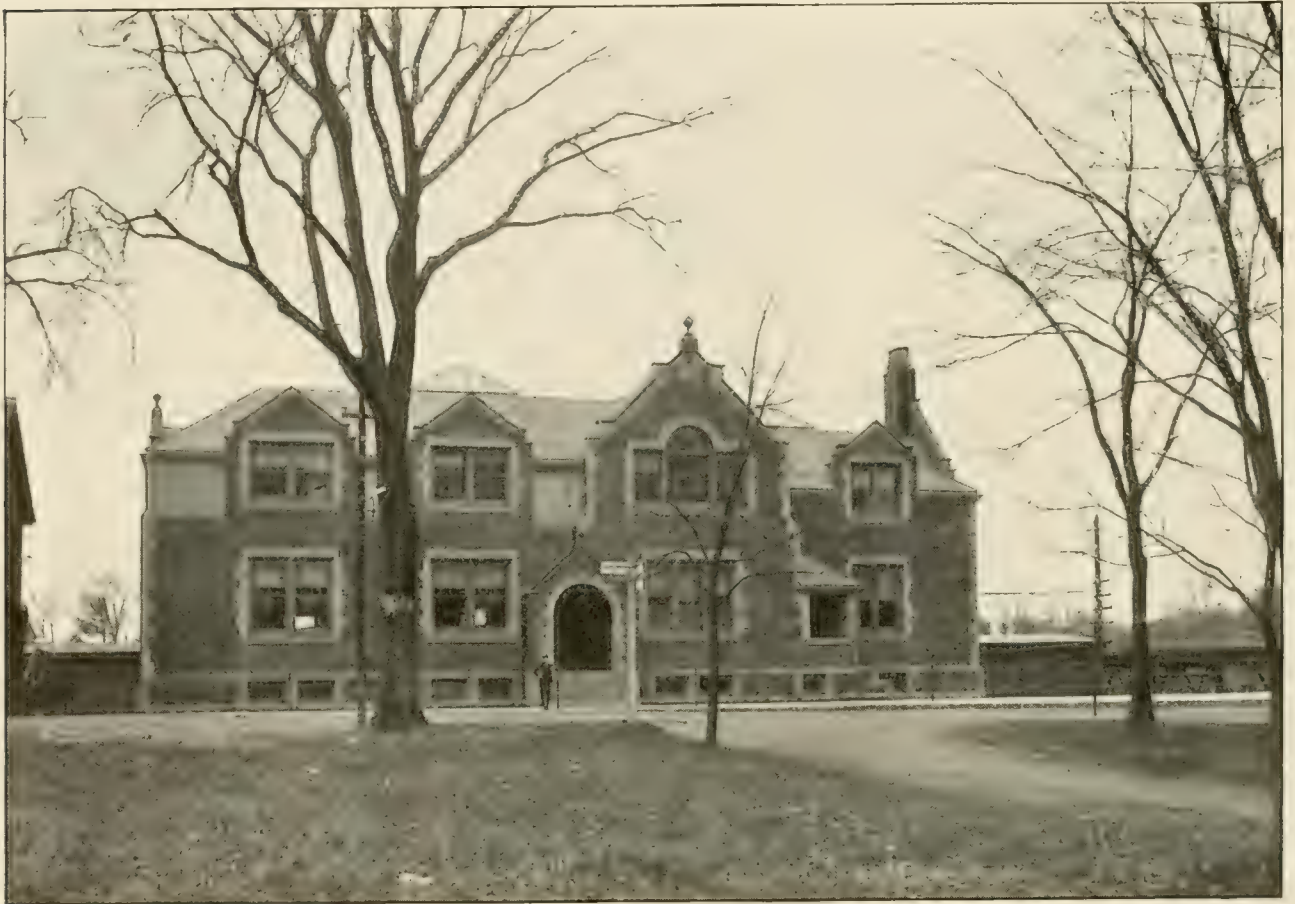
OFFICE BUILDING OF LUDLOW MANUFACTURING ASSOCIATES
