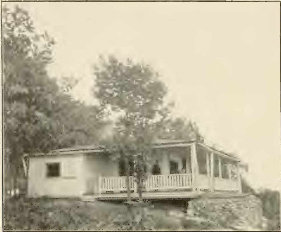
BUNGALOW OF F. L. BURR ON FACING HILL ROCK
