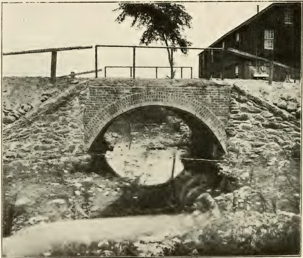
ARCH BELOW H. I. CARVER'S MILL
