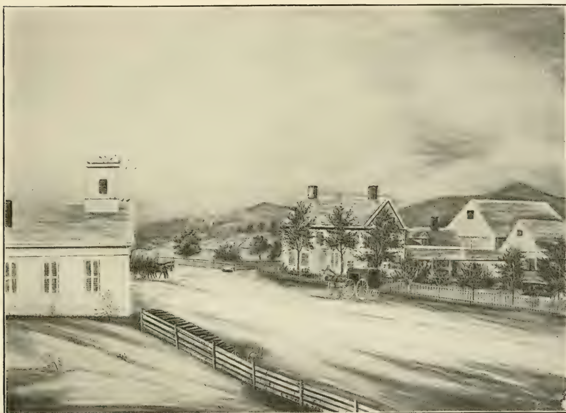
METHODIST CHURCH, JENKSVILLE Built in 1847. Removed in 1863 to Warren
