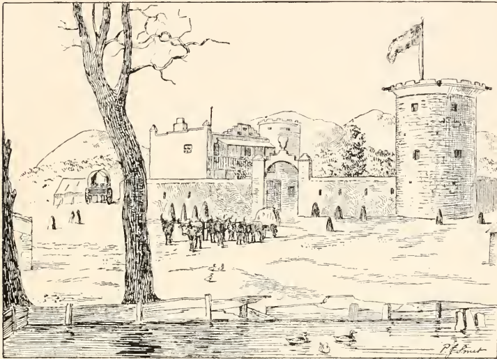
CASTELLATED RESIDENCE IN ZOUTPANSBERG.
