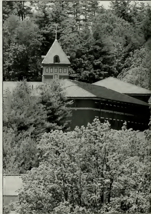
New Building • The new Living and Learning Center located off Bodenheimer Drive contains both a residence and an academic wing. The building was opened in the spring of 2003 and housed the Interdisciplinary Studies Department.
