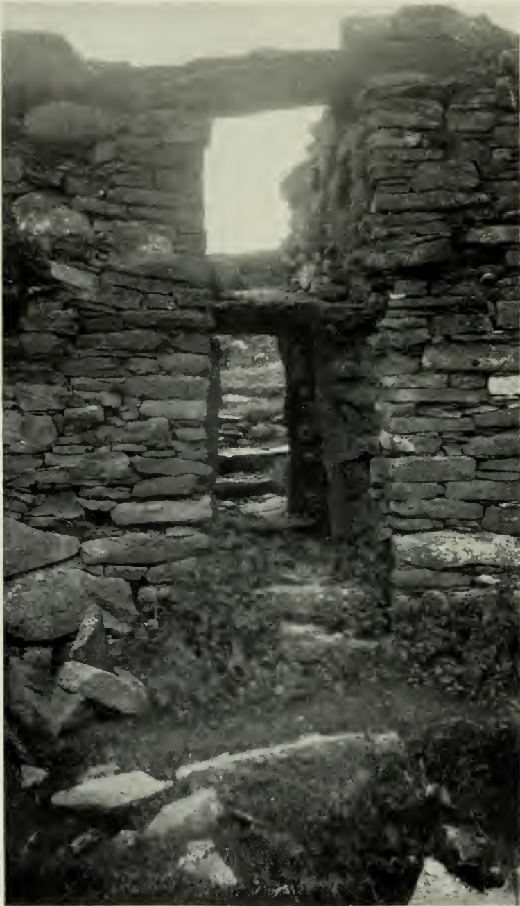
PLATE XVIII.—Broch, Ousedale Burn: entrance from interior (No. 204).
