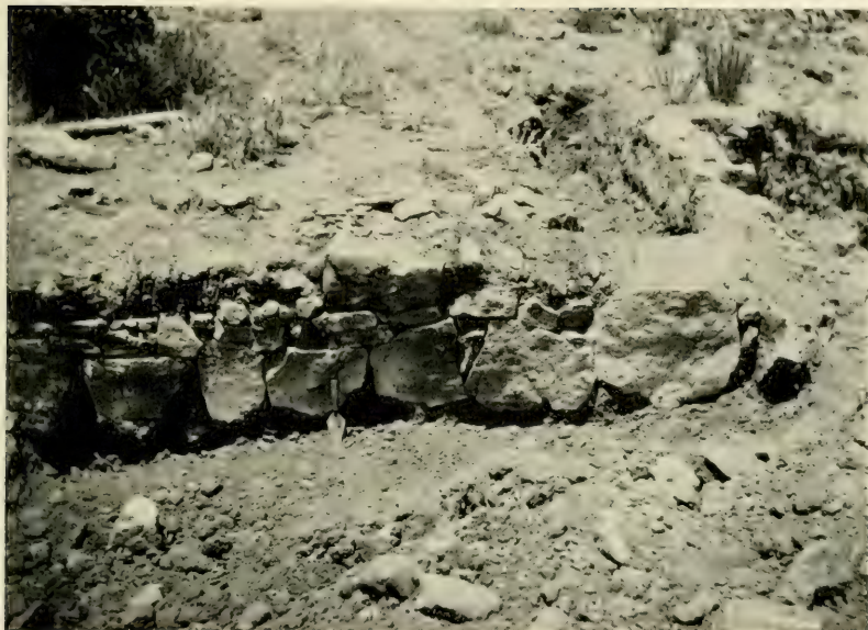
1. Showlow. Basal part of an old wall showing the use of large blocks surmounted by small stones in poorly constructed horizontal courses.
