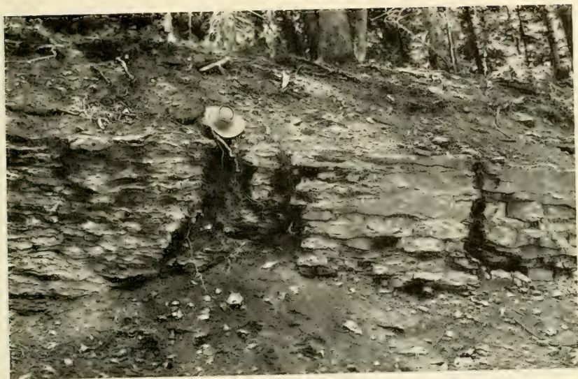
1. ROAD CUT IN SANDIA MOUNTAINS, FIR-SPRUCE ZONE, SHOWING SOLUTION-WIDENED JOINTS IN LIMESTONE CONTAINING LIMONITIC CLAY
