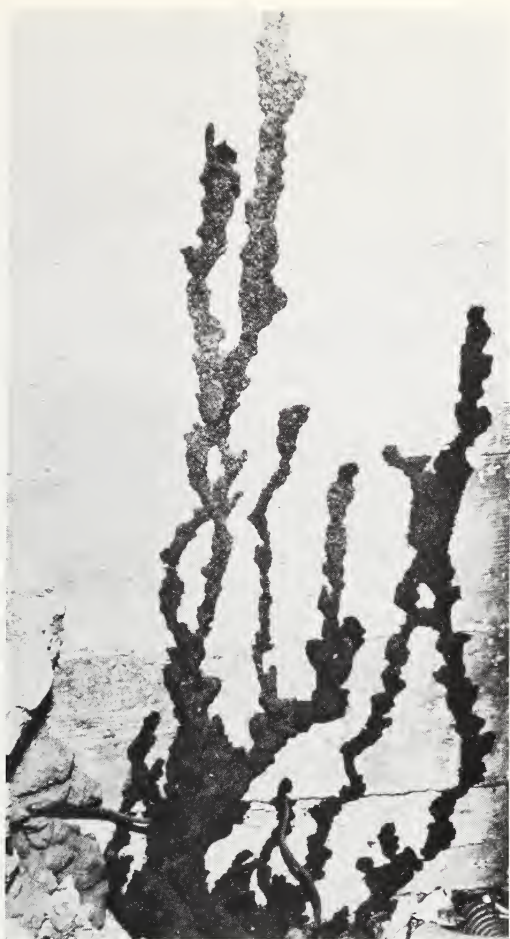
FIGURE 30.—Earthenlike tubes built over cement foundation by western subterranean termite ( Reticulitermes hesperus ).
