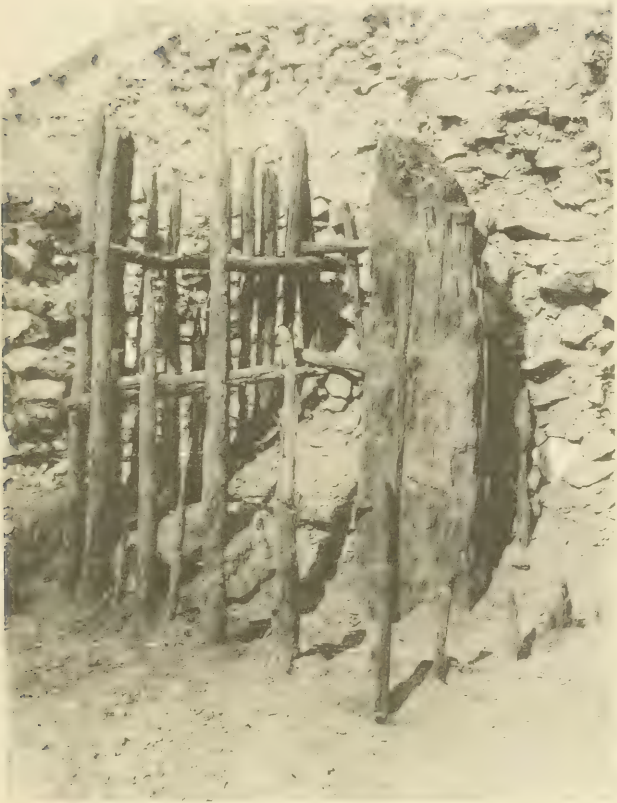
CEDAR BEAMS AND POLES TEMPLE OF QUETZALCOATL
