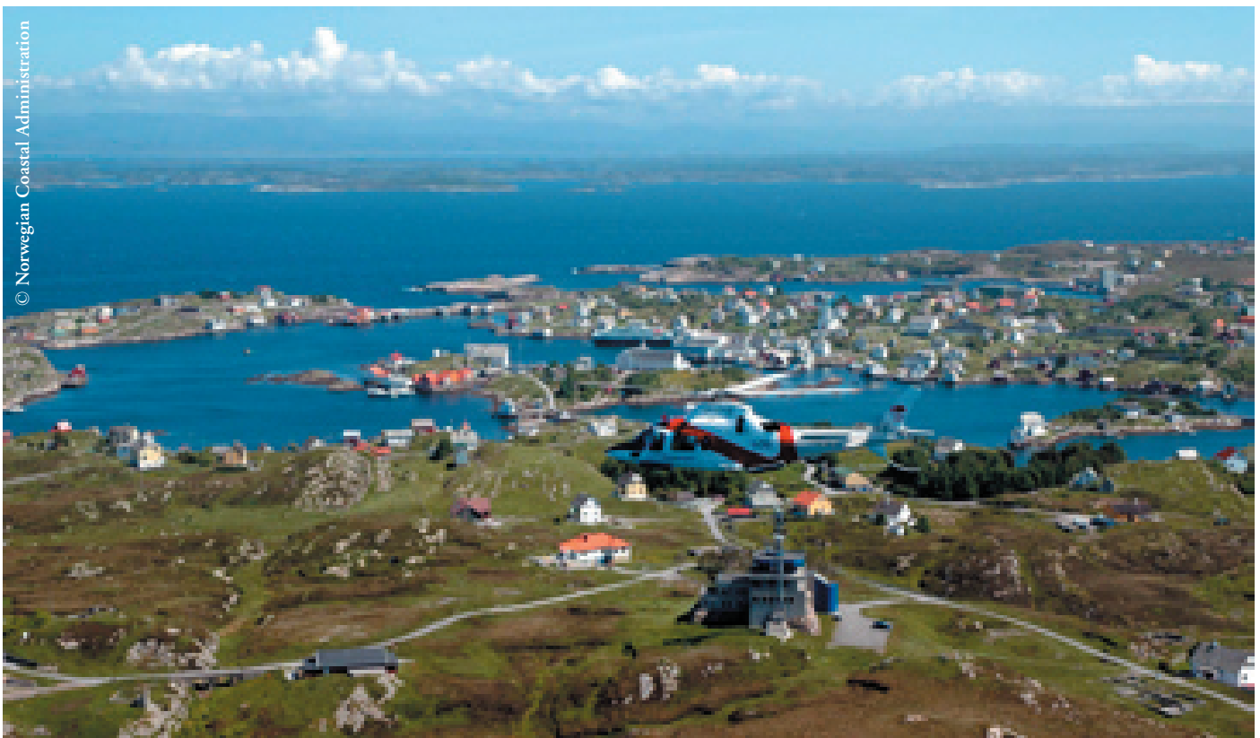
Figure 6.4 From the helicopter one can see the Fedje traffic control with the residential district of Fedje in background. Fedje traffic control controls one of the busiest traffic zones in Europe. In Europe only Rotterdam has a larger amount of ship traffic through the year than Bergen and the adjacent sea area.
