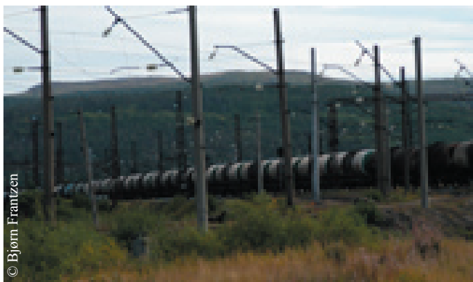
Figure 4.6 In 2004 more than 7 million tons of export oil was sent to Vitino and Murmansk by the October Railway (Moscow-Murmansk line). In 2010-2015 the expected growth of freight by rail to Murmansk will be 40 million tons a year. This train with oil tank cars was passing Kandalaksha in September 2004.
