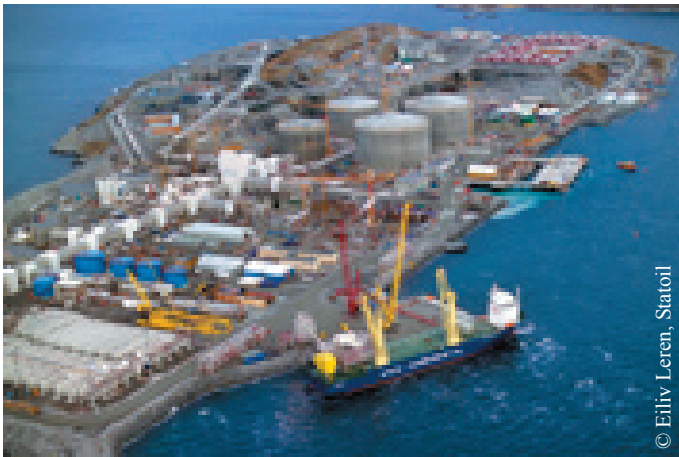
Figure 5.4 This is how the land installation of Statoil's Snøhvit project appeared at Melkøya, Hammerfest, in November 2004.
