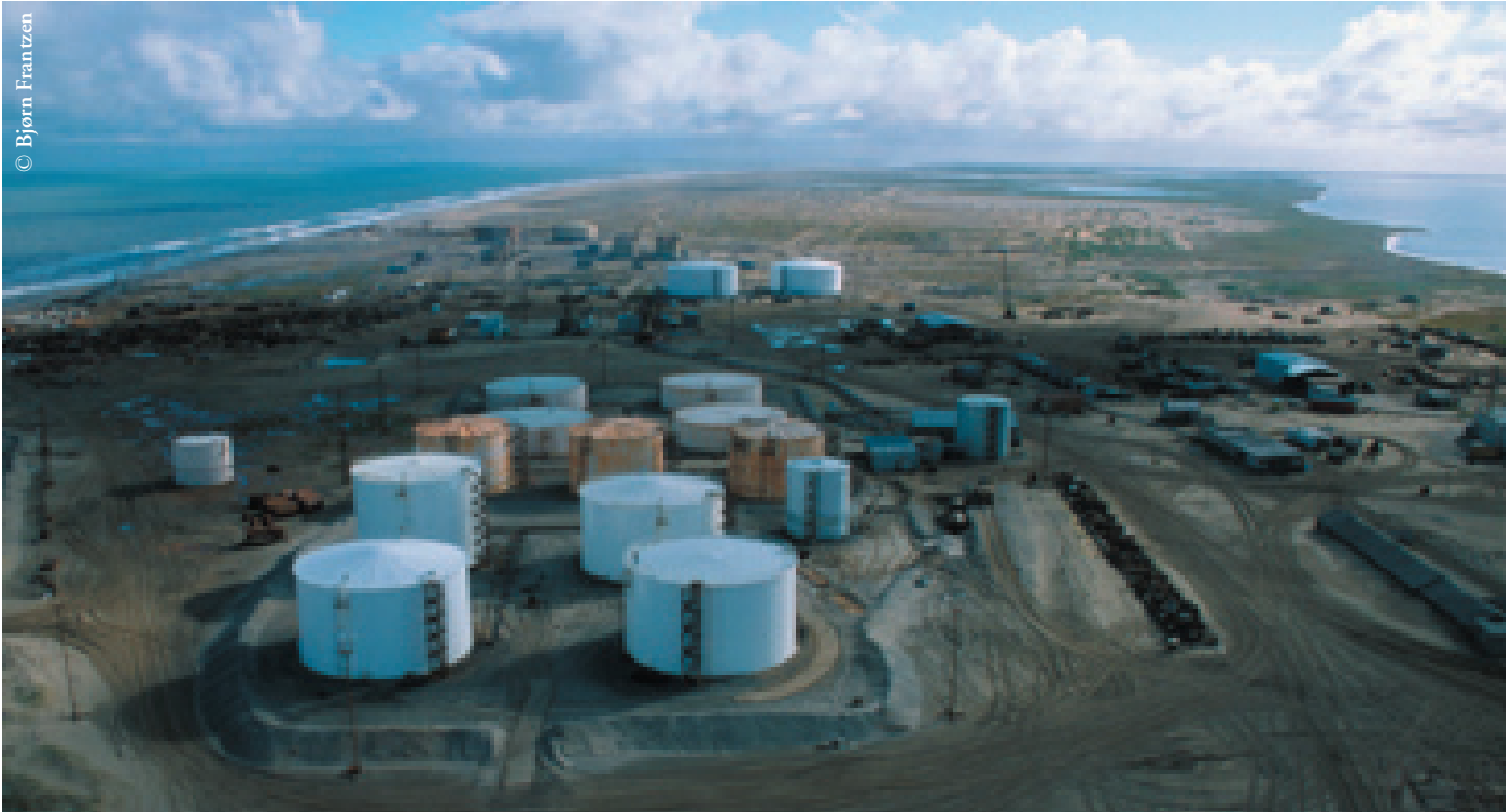
Figure 4.21 The Lukoil subsidiary Arktikneft is responsible for the extraction and shipment of oil from Kolguev. In recent years 80 000 to 100 000 tons of crude oil has been shipped annually from Kolguev, now only in the summer period from June to October.
