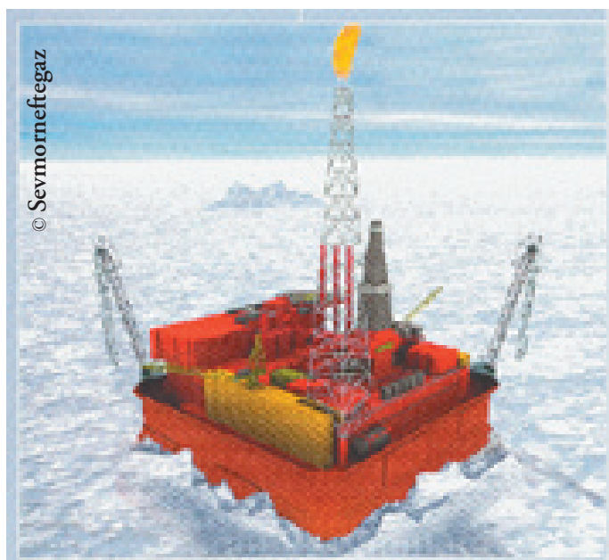
Figure 4.23 The Prirazlomnaya platform will be the first commercial oil production platform operating in the Arctic in an area that is ice covered six months a year. According to the plan, the platform will be towed to its position in the Pechora Sea during the summer of 2005 and the drilling will start late the same year. The platform is expected to export maximum 7.5 million tons a year.
