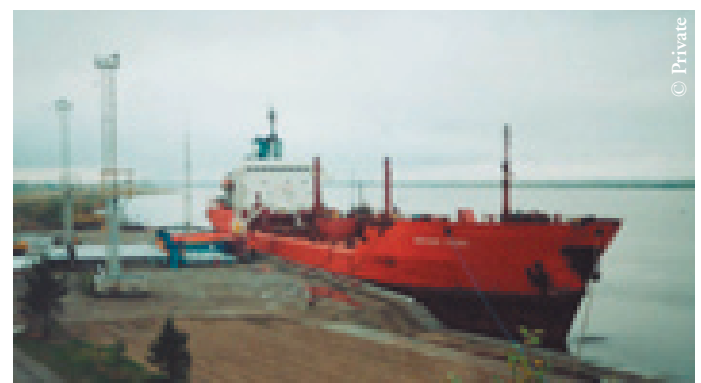
Figure 4.25 The Russian tanker Aleksandr Sledzyuk loading at Rosneft-Arkhangelsknefteprodukt Talagi oil terminal. This ship shuttles oil between Talagi and the FSO Belokamenka in the Kola Bay.
