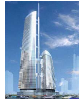
Federation Building Moscow, Russia, under construction
