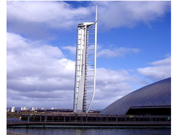
Millennium Tower Glasgow, Scotland, 2001
