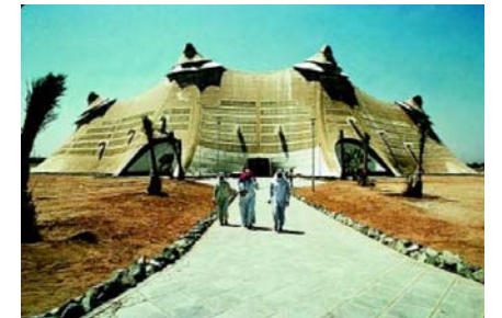
Gymnasium in Jeddah, Saudi Arabia Jeddah, Saudi Arabia, 1980
