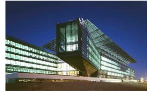
Endesa Headquarters Madrid, Spain 2004
