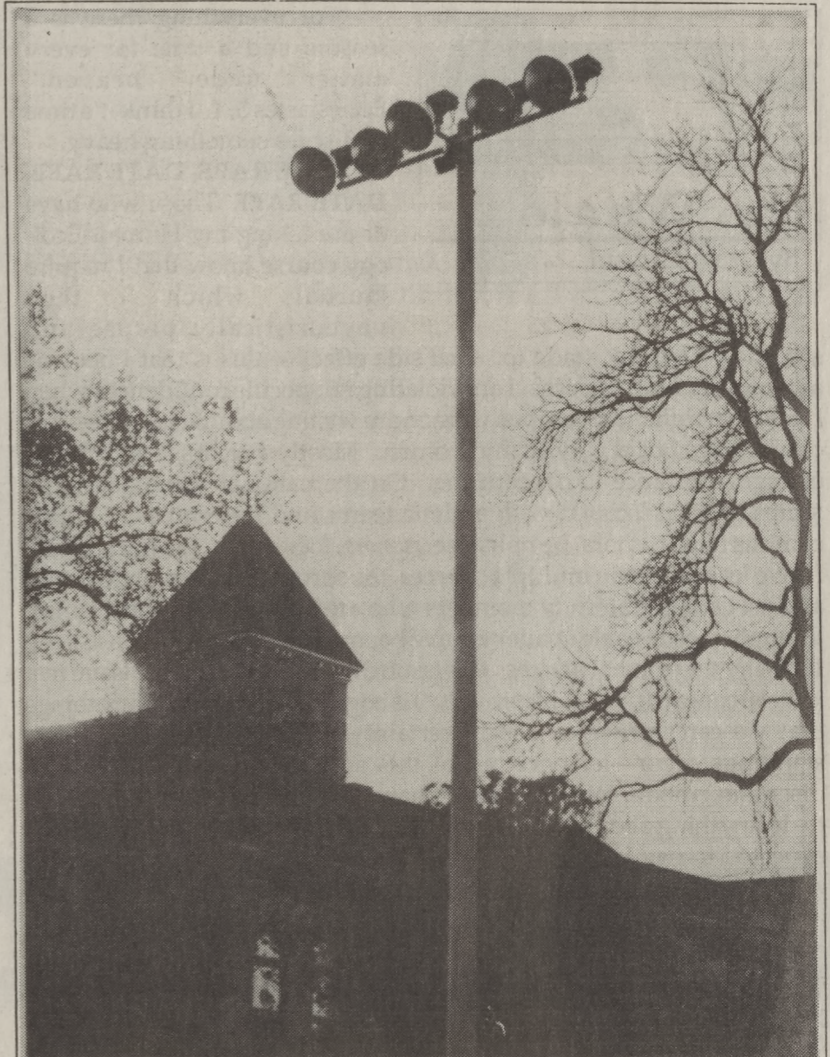
The new tennis court lights being installed
