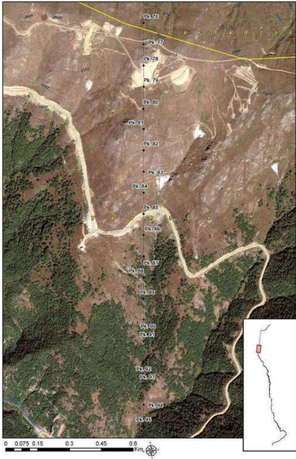
Figure 86: Kajaran-Agarak highway alignment (Tranche 4, Lot 2), Tashtun village, Pk 7.7 – Pk 9.5
