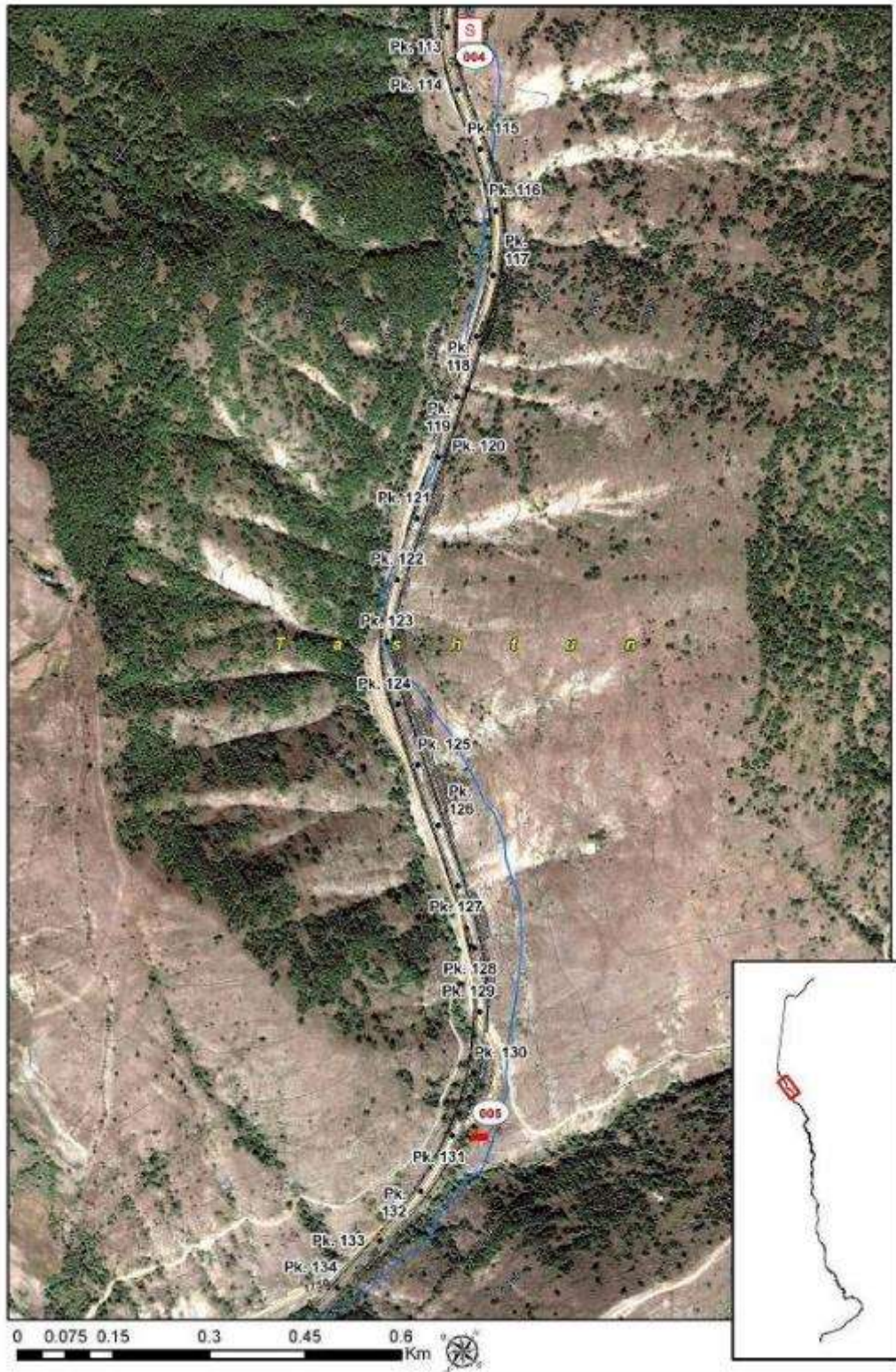
Figure 90: Kajaran-Agarak highway alignment (Tranche 4, Lot 2), Tashtun village, Pk 11.5 – Pk 13.4
