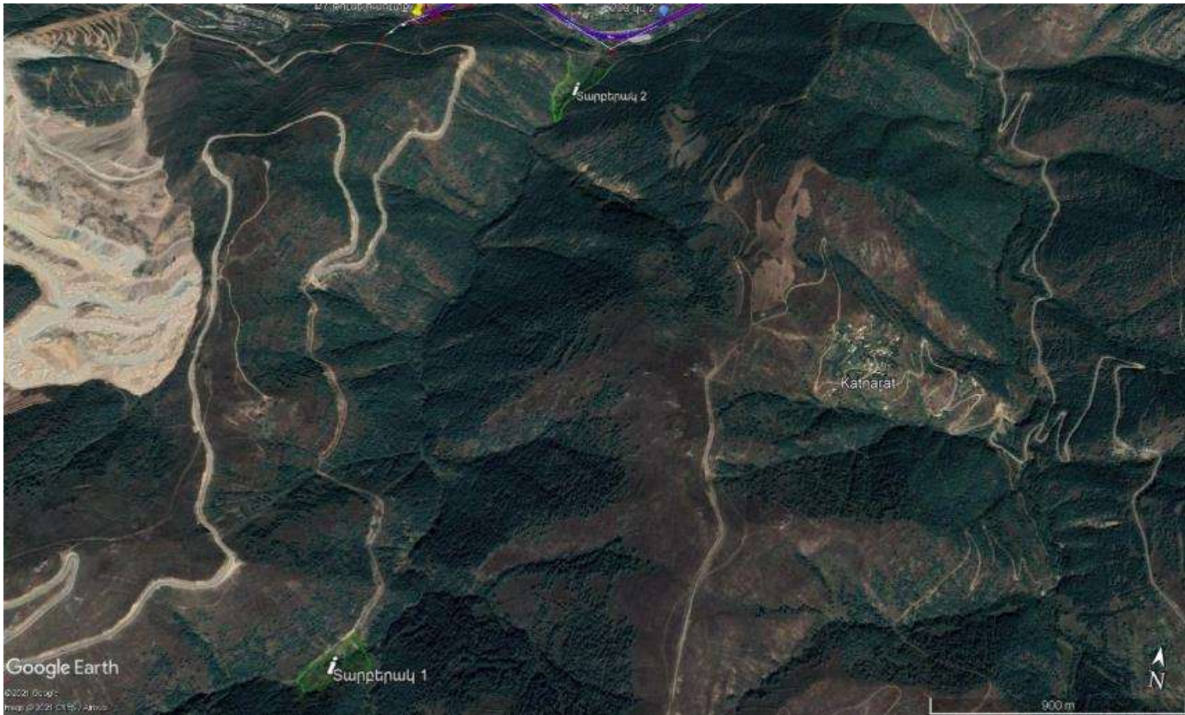
Figure 123: Photo of the recommended area of the dumps with Google Earth program
