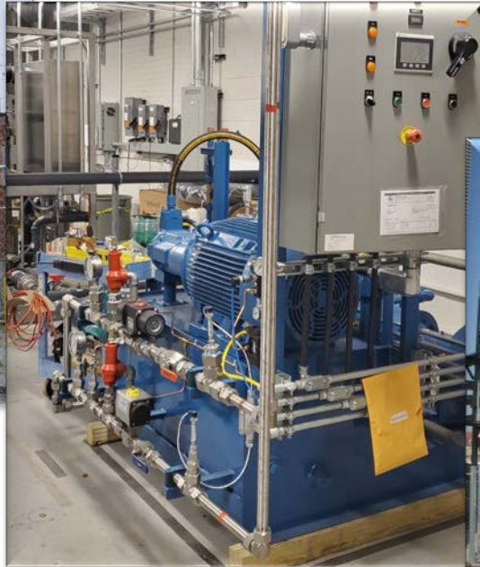
CO 2 heat pump & power cycle
