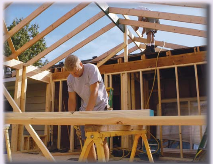
New home construction
