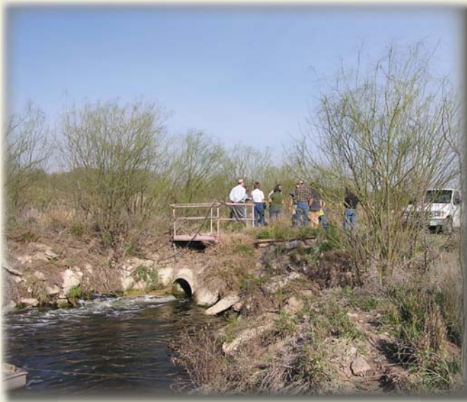
Wastewater outfall, Mission
