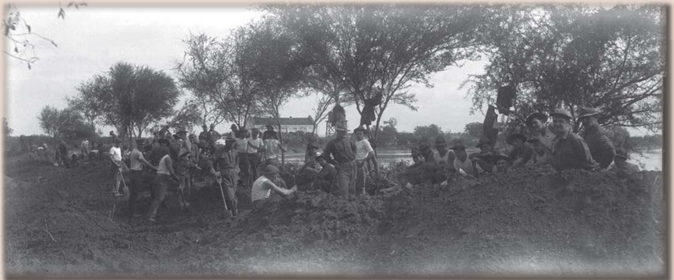
Soldiers working on levee, circa 1917
