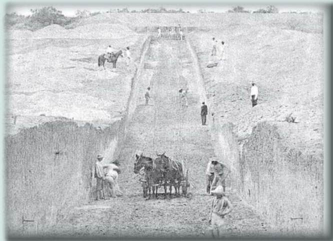
Canal-building in the 1900s
