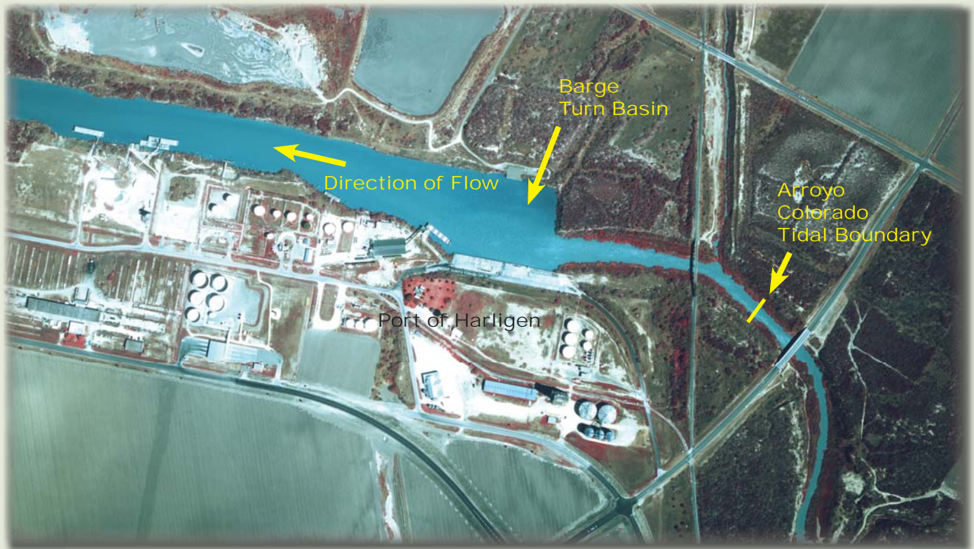
The Arroyo Colorado was widened and deepened to create the Barge Turn Basin at the Port of Harlingen immediately downstream of the tidal boundary
