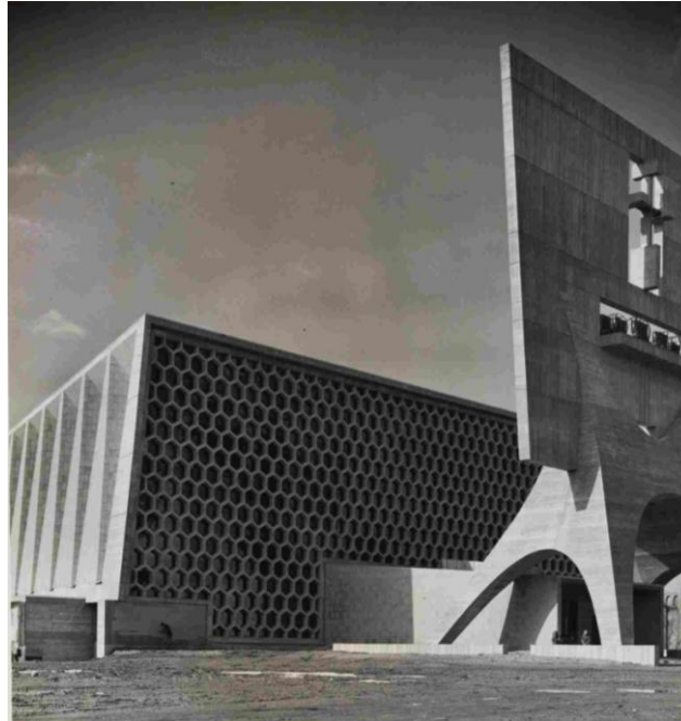
Figure 1 Photograph of Marcel Breuer's St. John's Abbey Church, Collegetown, Minnesota, United States (1953-1961). General view from the north-east showing hexagonal tracery of north wall set with stained glass, atrium wing, and bell-banner. Photo courtesy of Marcel Breuer Papers, Special Collections Research Centre, Syracuse University Libraries.
