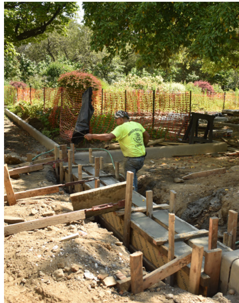
Irrigation work in the South Garden
