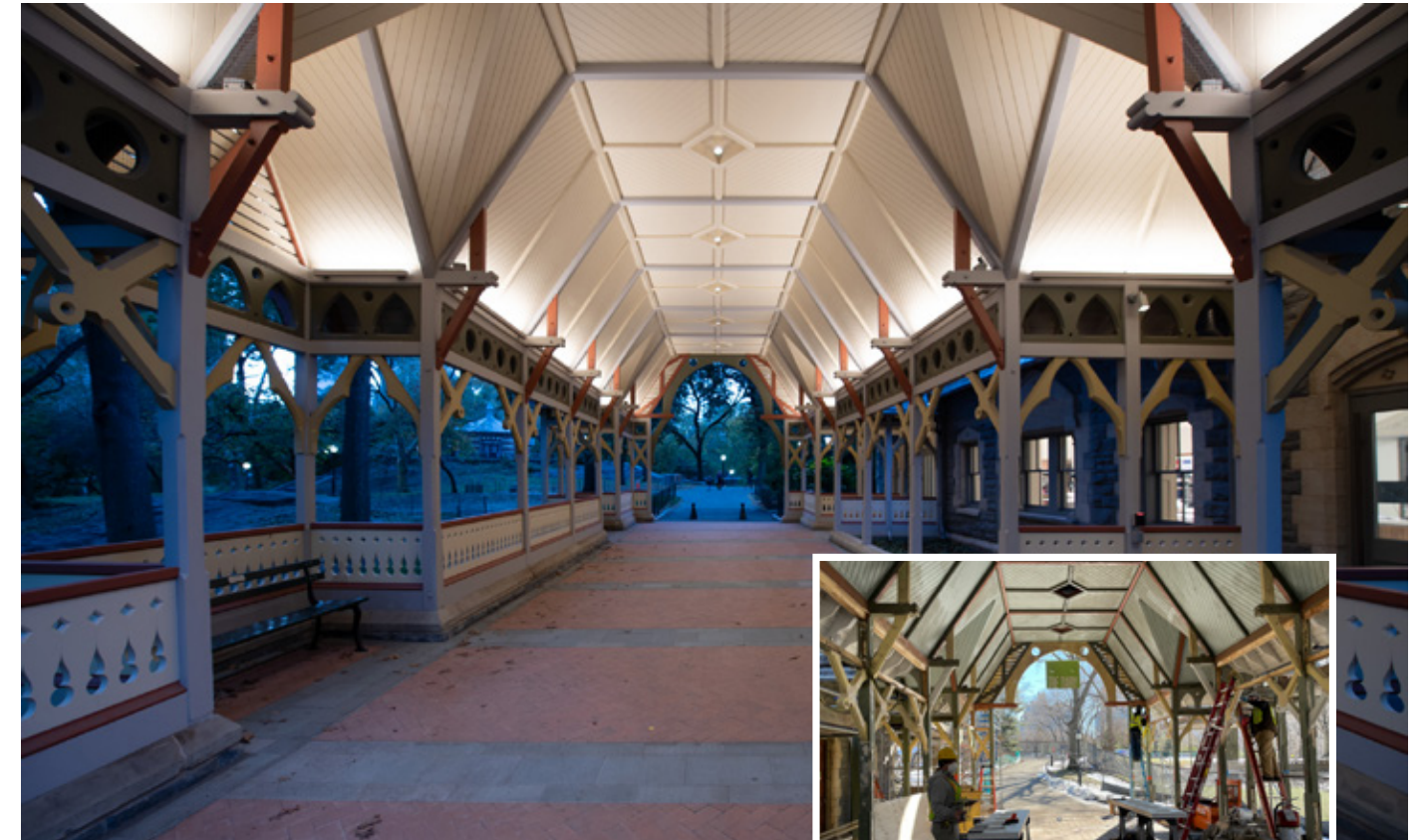
The historic loggia, pictured here post-restoration, was repaired as part of the comprehensive renovation; inset: construction underway.
