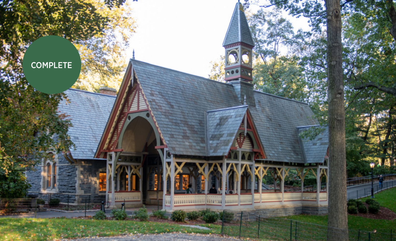
The completed Dairy
