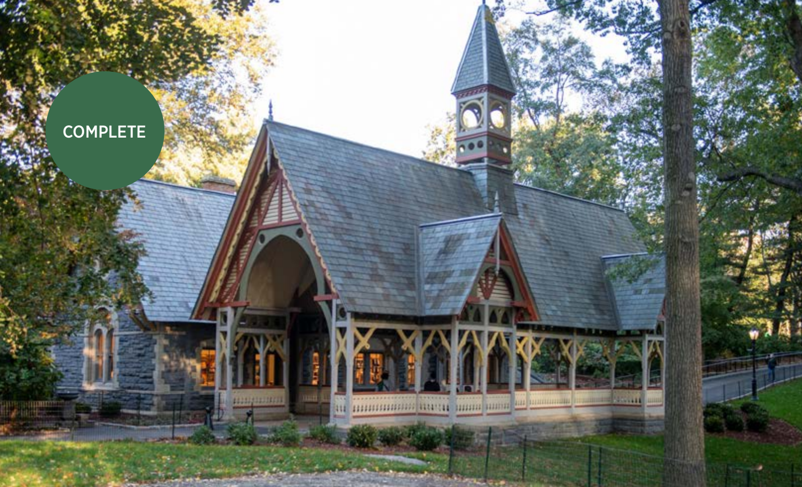
The completed Dairy
