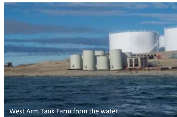
Shore access at West Arm Tank Farm.
