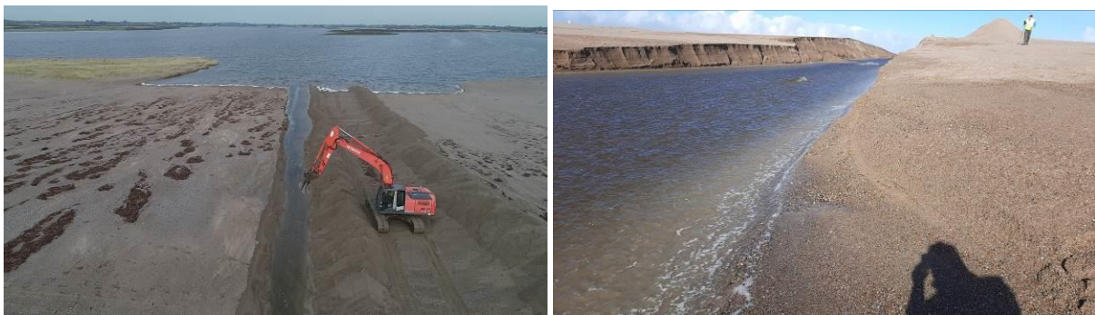
Plate 5 The cut being made at Southern end of Lady's Island lake in March 2021 (left) and completed cut (right).
