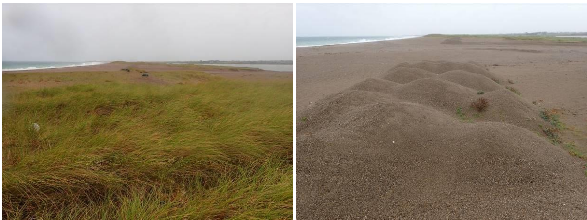
Plate 9 Sand dune system associated with the barrier beach to the east of the 'cut' at Lady's Island Lake (left). This part of the due system is subject to mush disturbance by excavation and mechanical movement of sand (right).
