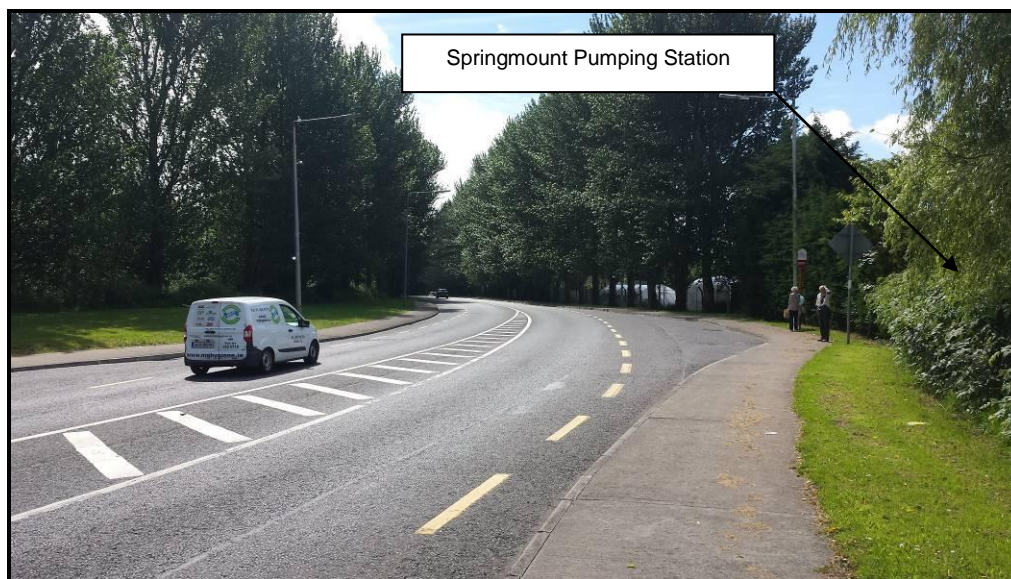
Plate 1: View of Springmount Pumping Station at the Spring Roundabout.
