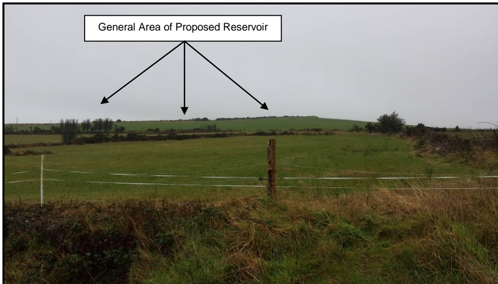
Plate 14: View of the area of the proposed reservoir looking from Robert's Cross towards Byrne's Cross (hidden behind the hill). The exact location is yet to be determined.
