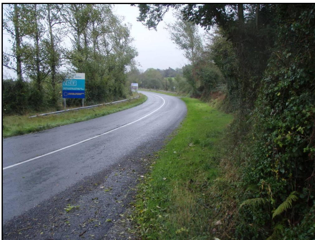
Plate 8: View of the R674 looking east. This road was built as part of the Dungarvan to Youghal trade route in the early 19 th century, and has been widened in modern times. The pipeline will be laid within the road.
