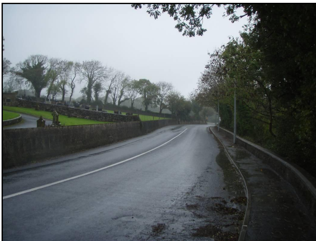
Plate 10: View of the R674 at Shanacloon. The graveyard is to the right. Note the retaining walls where the road appears to have been widened. The pipeline will be laid within the road.
