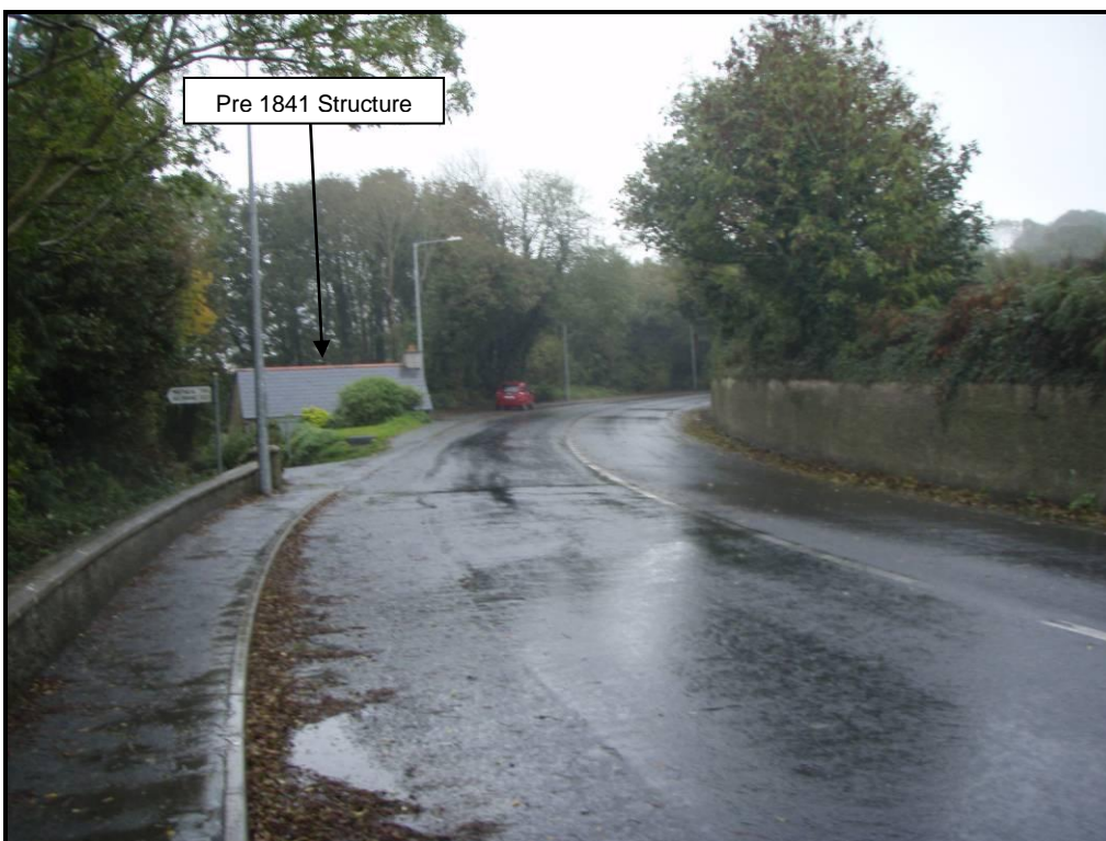
Plate 12: View of the R674 at Shanacloon. The Graveyard RMP WA036-008002 is to the right, out of picture. Note the recently restored structure which is shown on the 1841 Ordnance Survey. Holy Well RMP WA036-007 lies among the trees to the left. The pipeline will be laid within the road.
