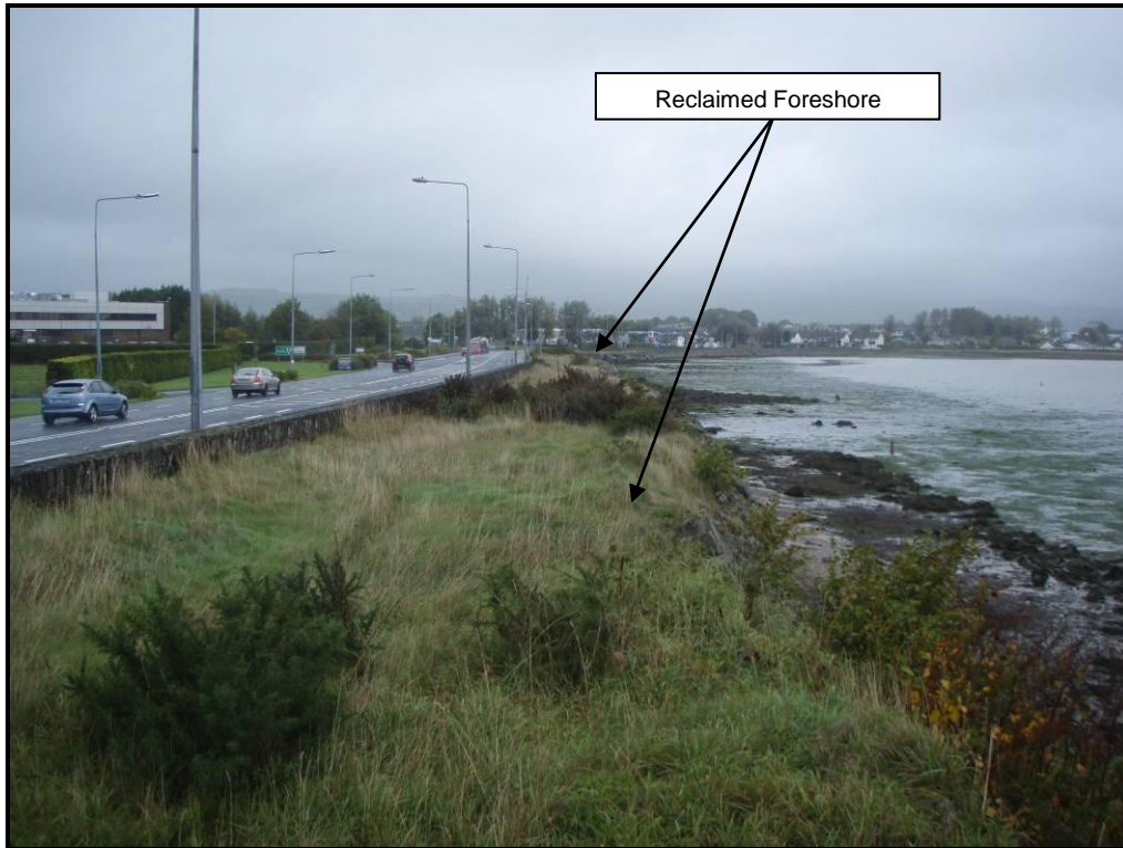
Plate 3: View of the N25 Dungarvan Bypass Youghal Road section, looking north showing reclaimed foreshore. The pipeline will be laid in the north bound road verge.
