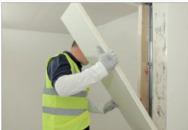
Figure 4 Window reveal installation
