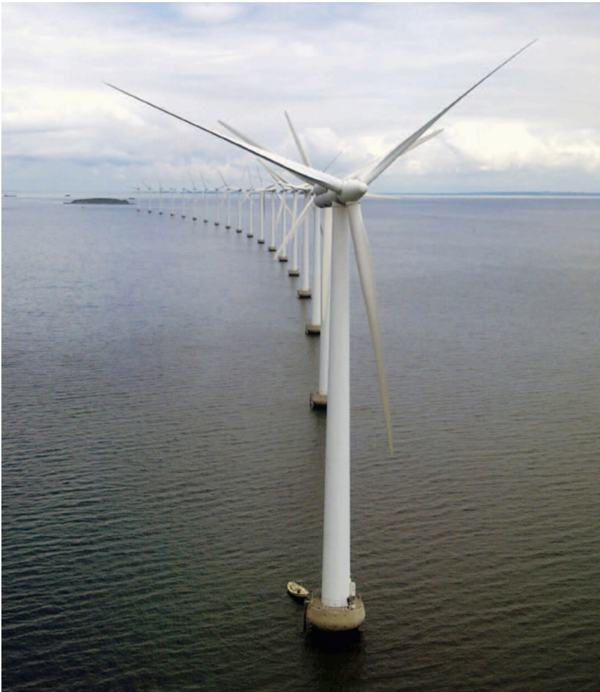
16-3. Offshore wind farm.
