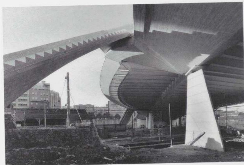
Underside of bridge during construction
