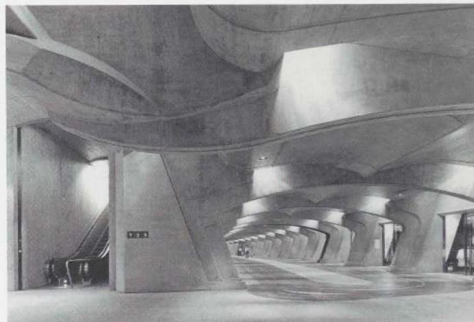
Lower commercial level and subway connecting element between platforms
