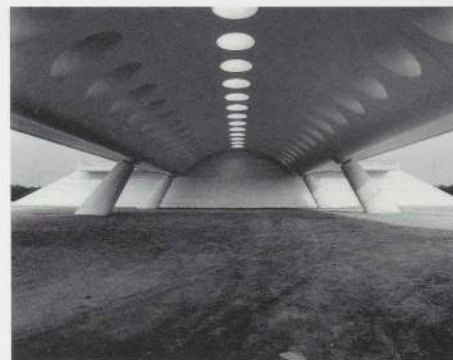
Underside of viaduct
