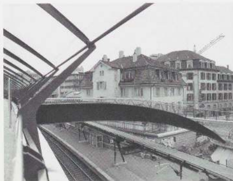
View of footbridge (Falkensteg)
