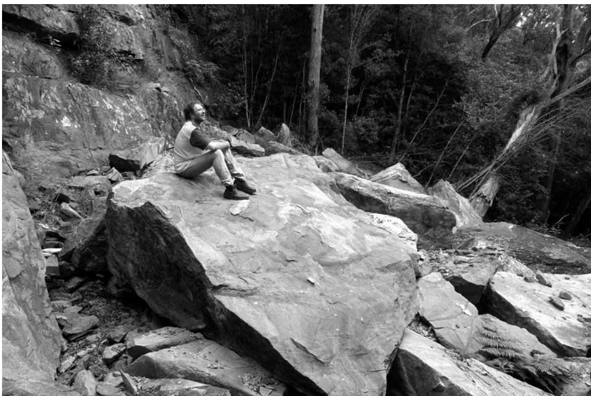
David Burgess inspects cliff fall damage at the Dendrobium Colliery in the Metropolitan drinking water supply catchment near Lake Cordeaux storage. Photo: K. Muir.
