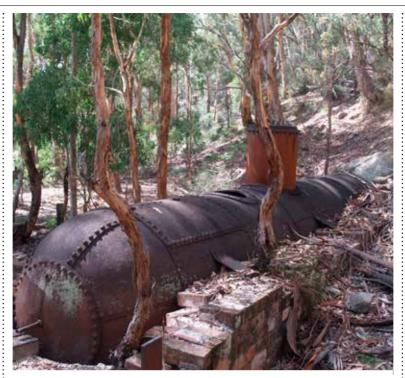
Boiler for aerial ropeway winding engine, New Hartley Oil Shale Ruins Image: K. Muir
