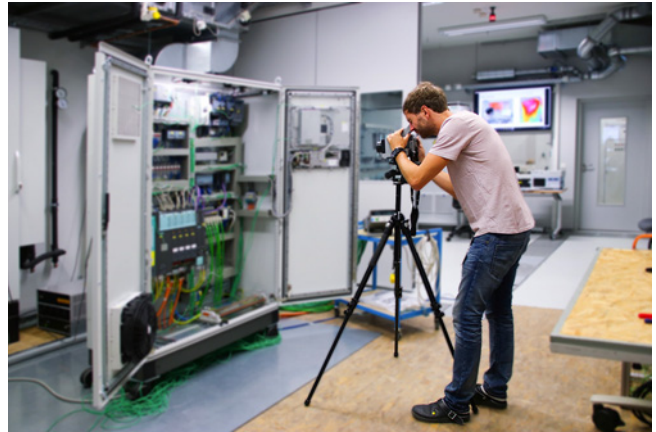
WKC - Test laboratory - Heat measurement
