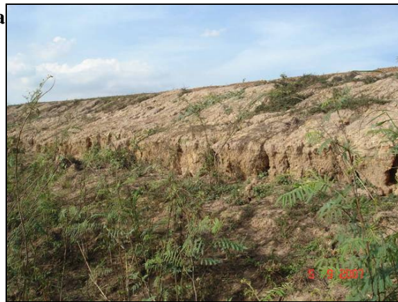
Figure 3. Illustration of Wave Erosion on a Section of RN 8 in Prey Veng.
