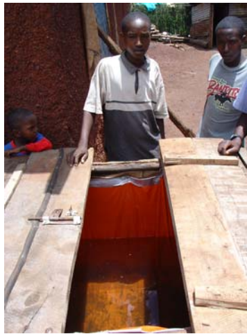
Figure 9. Home-made water reservoir in Kirehe Sector in Rusumo District.
