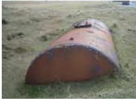
Tank removal before
