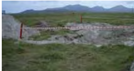
Tank removal during
