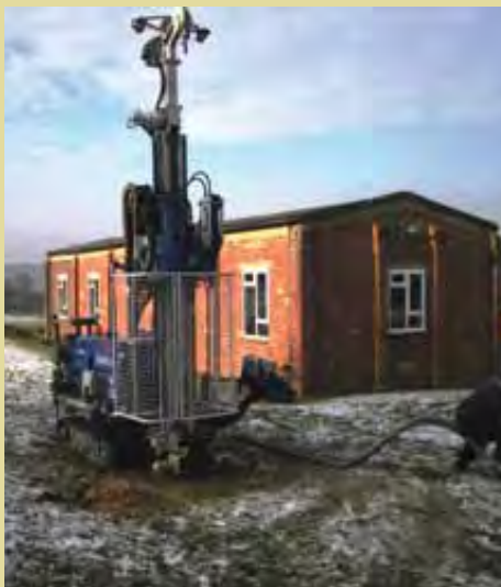
Drilling rig for ground coil, Crowborough Camp © Kevin Hoare
