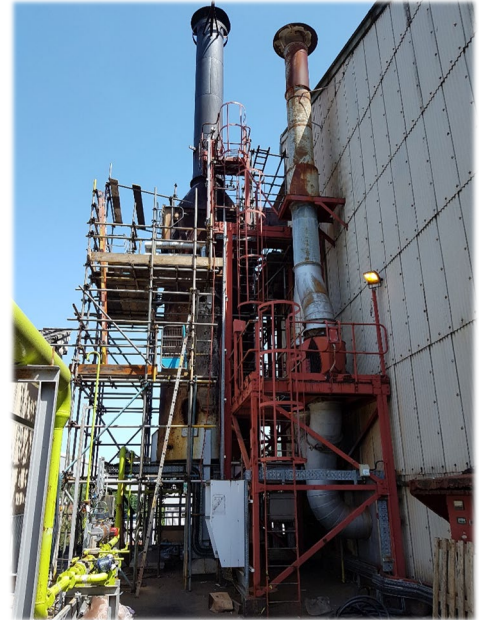
Example hydrogen heater that will either be replaced by conventional plant or resilient fuel switching plant.
