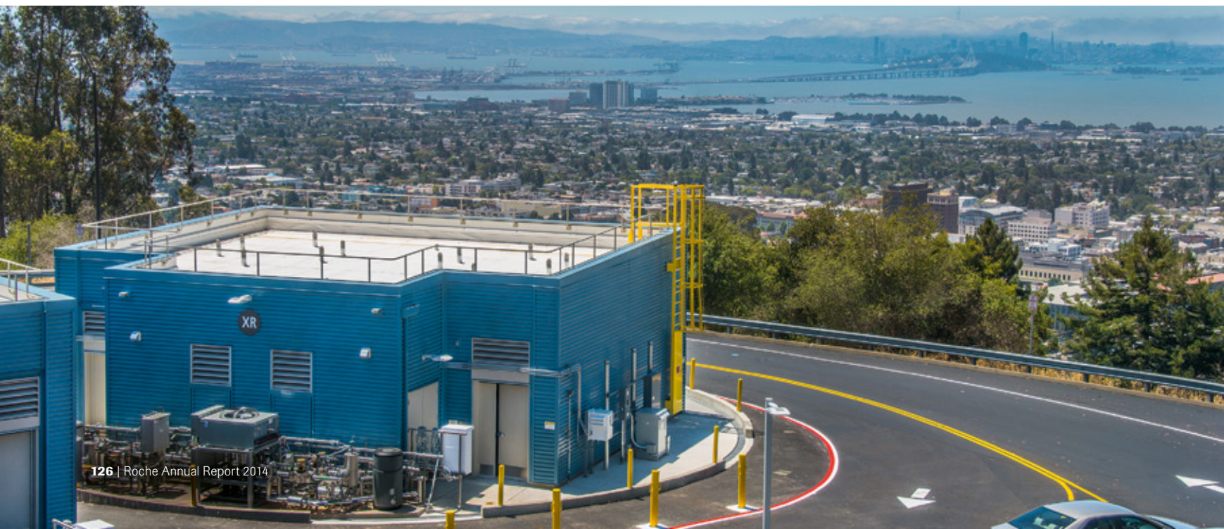
The FLEXLAB provides state-of-the-art technology to optimise energy efficiency of new buildings, helping to save energy and water.
